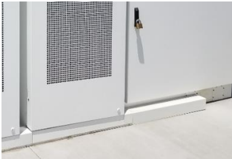
Figure 8-5 Installed wireway flush in bottom of Powerpack 2 enclosures
