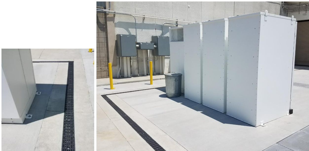
Figure 12-6 Trenches for drainage
