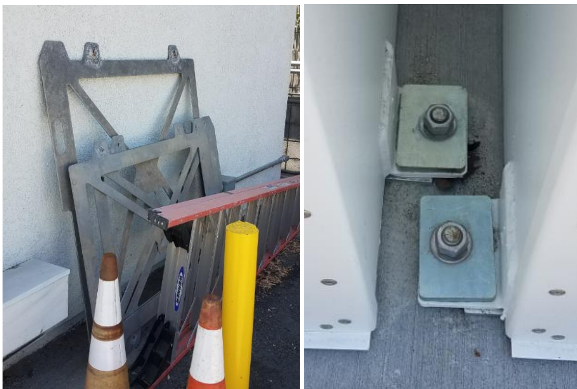
Figure 12-5 a) Mounting templates, b) mounting feet with seismic plates
