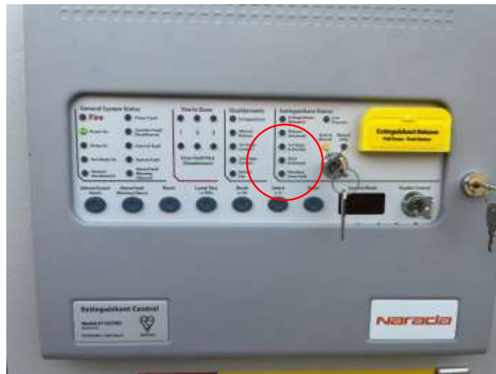
Fig. 6-4: FSS Control Panel Auto/Manual Switch (For reference)
