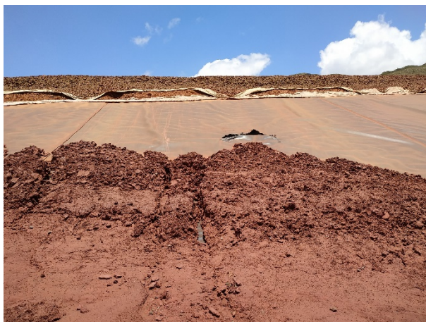
Photo 6: Perforation géomembrane (godet)
