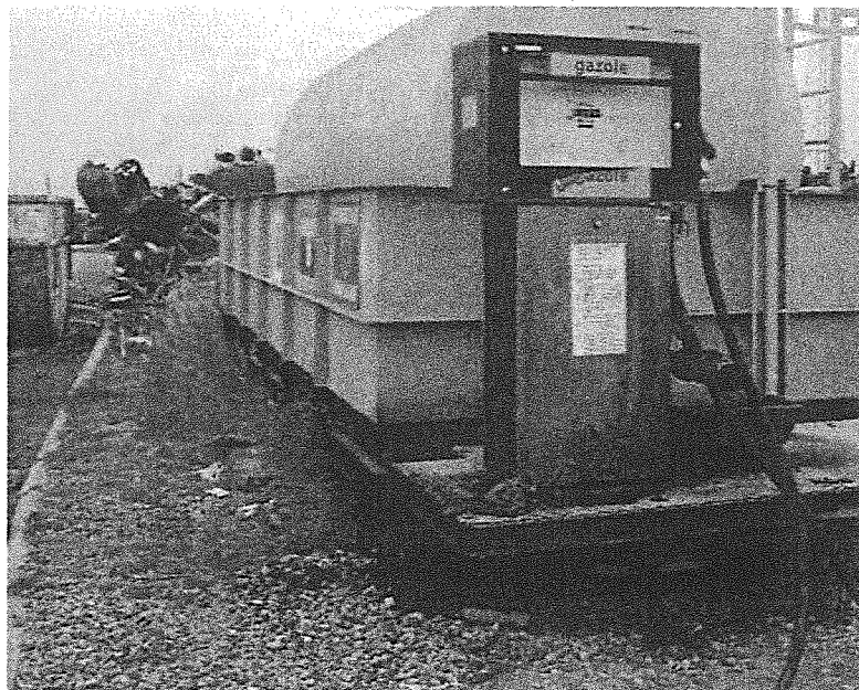
Image 9 – Installation de distribution de gasoil
