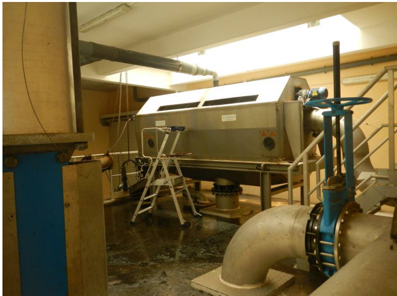
Figure 15 : Photo Soproner 2013 – Tamis
