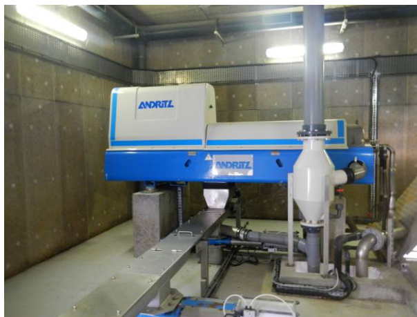
Figure 21 : Photo Soproner 2013 – Centrifugation
