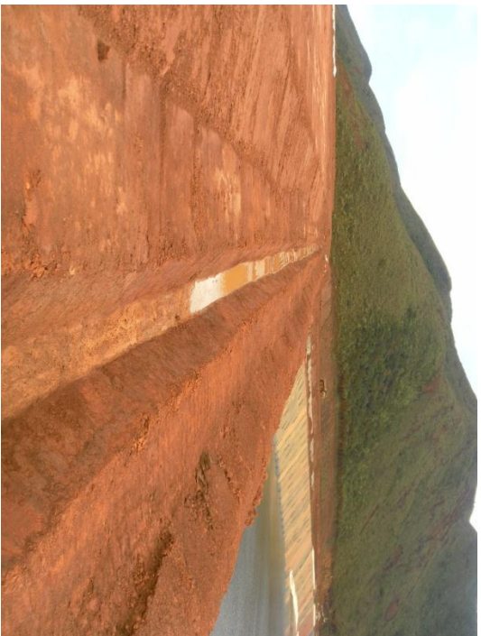
2.2.b - S1 1A Ditch water ponding
