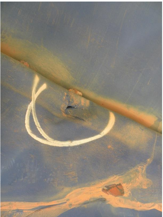
12.1.b Liner hole to be repaired
