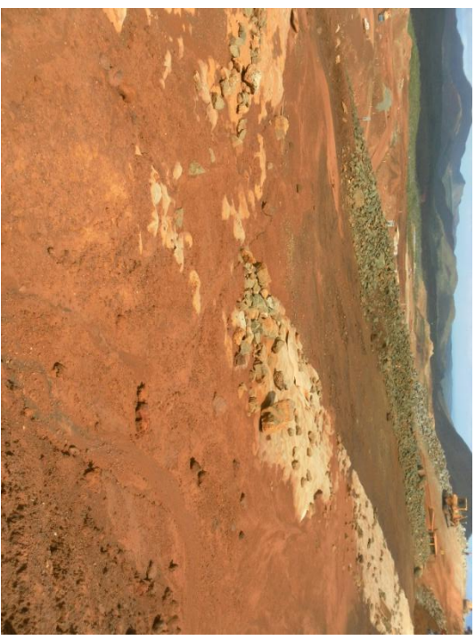
6.3. a S2 Limonite erosion to chimney drain hole
