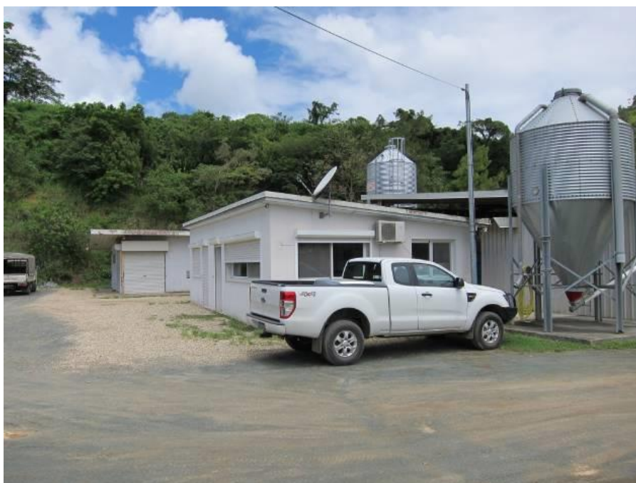
Figure 15 : Bureau/Accueil - Photo Soproner
