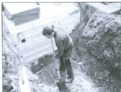
Pose station TOPAZE type T50
