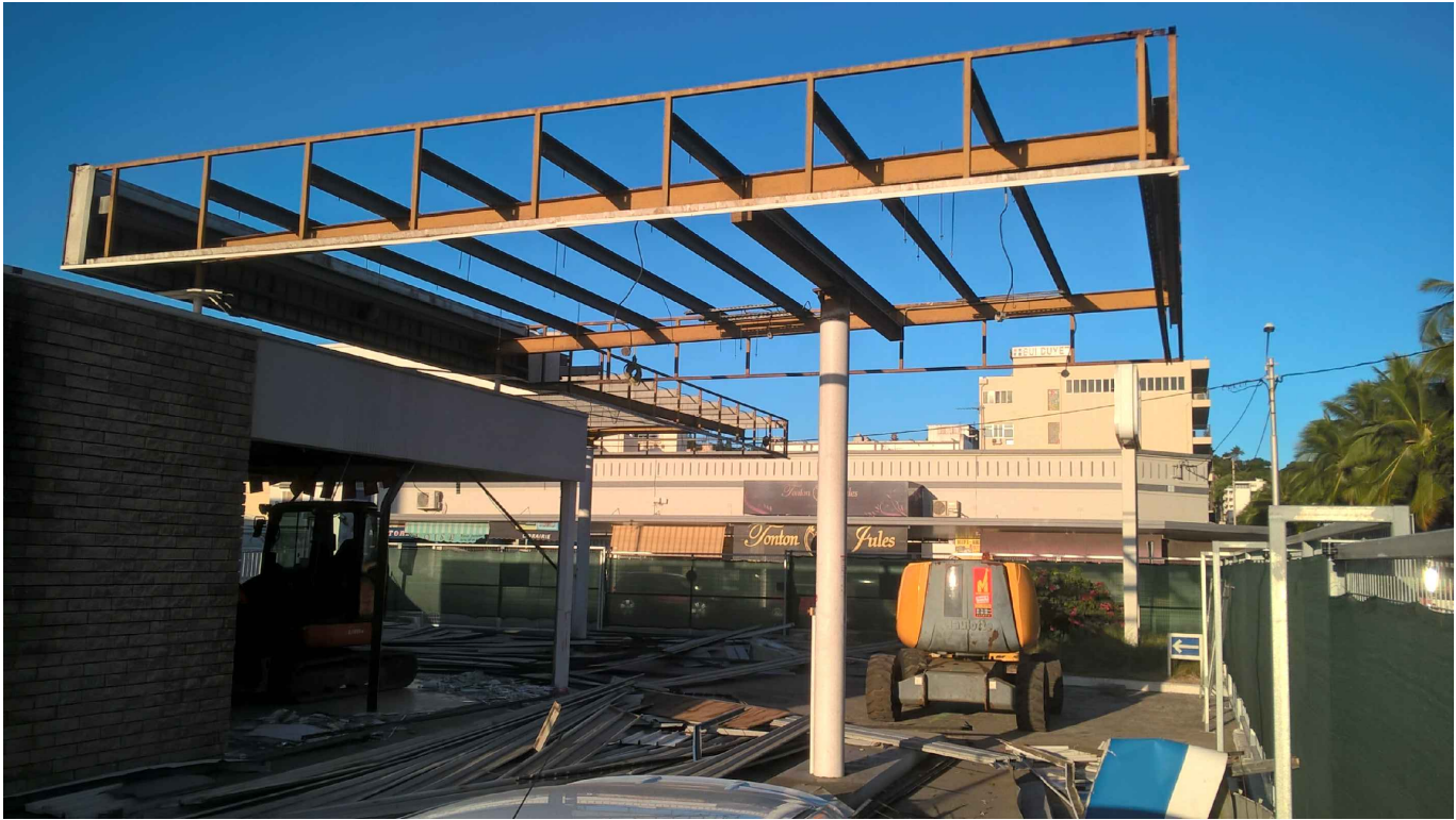
MID-DEMOLITION VIEW EAST OF CANOPY
