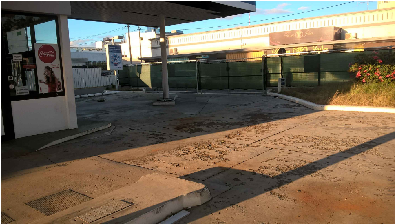
PRE-DEMOLITION VIEW NORTH-EAST
