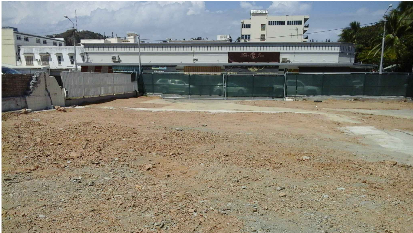
POST-DEMOLITION VIEW EAST ONSITE
