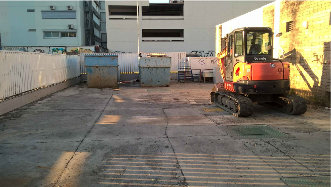
PRE-DEMOLITION UST FARM AREA
