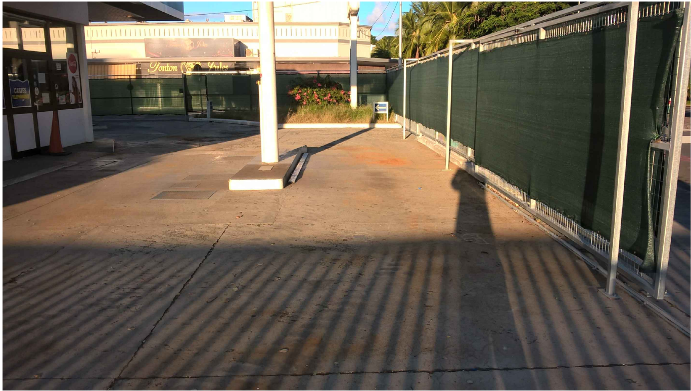
PRE-DEMOLITION VIEW EAST
