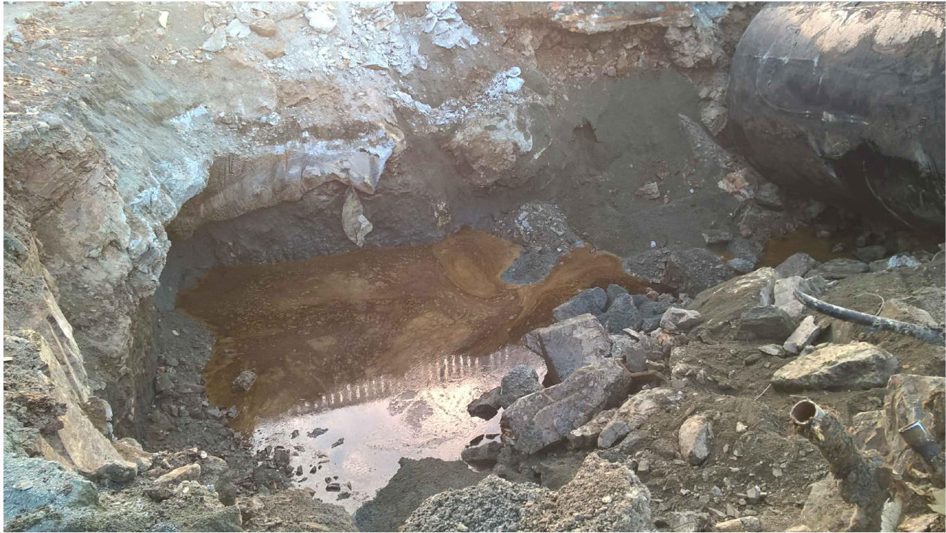
EXCAVATION EX01 MID-UST REMOVAL
