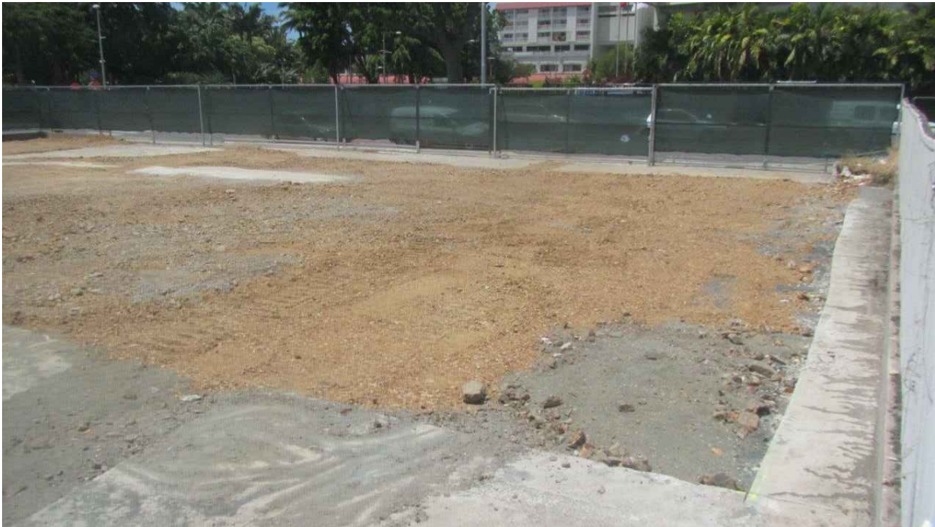
POST-DEMOLITION VIEW NORTH-WEST TO SOUTH-WEST
